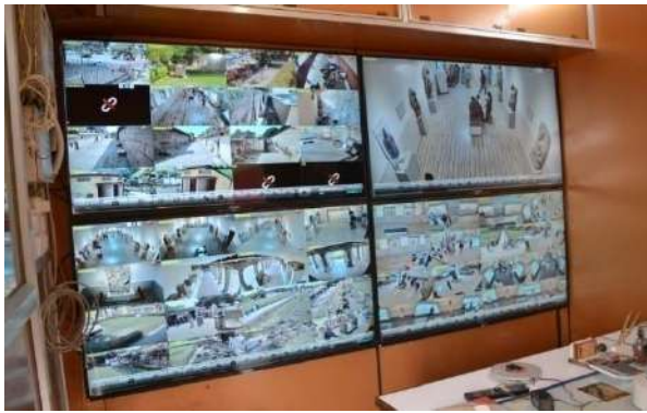
Monitoring unit of Installed CCTV Cameras
