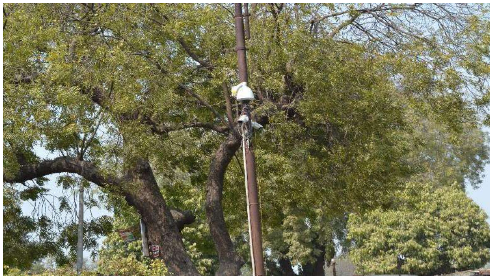
Installation of CCTV Cameras at the site.
